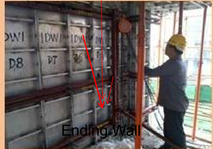
Ending Wall 墙模紧固背楞
