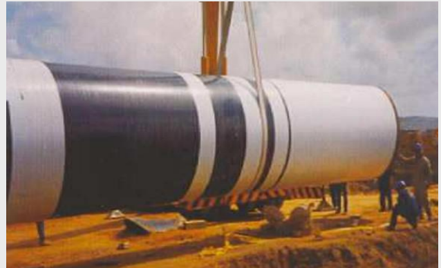
POLYKEN Line Travel Coating System
