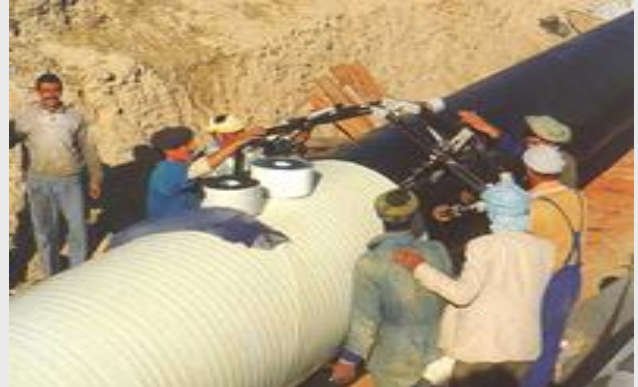
POLYKEN Line Travel Coating System
