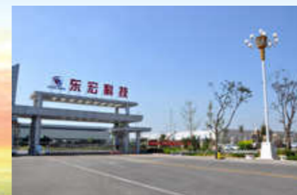
△ The South Plant of Donghong has been built and put into service which represented the development of Donghong enter into a new era.
